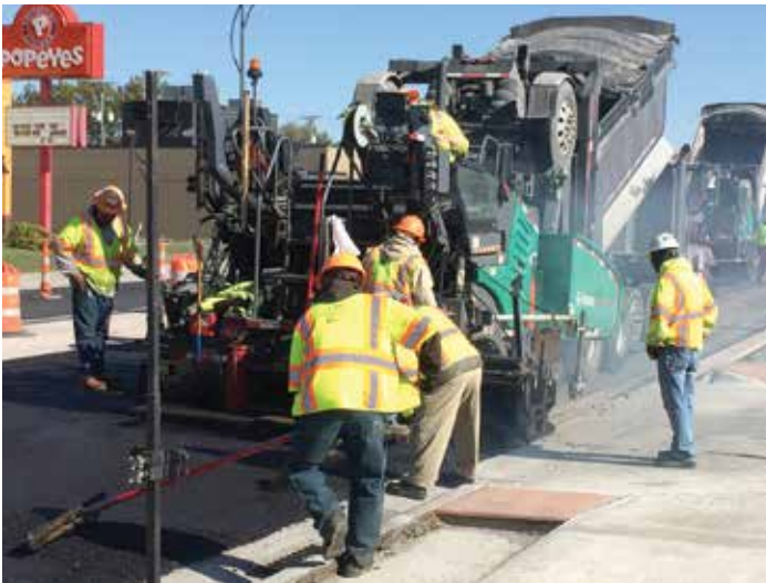
Omni Engineering crews paving final surface of West Broadway in October.
