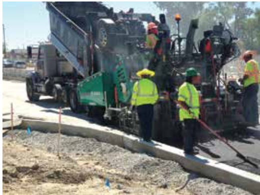
Omni Engineering paving crew placing the Perpetual Pavement base course.
