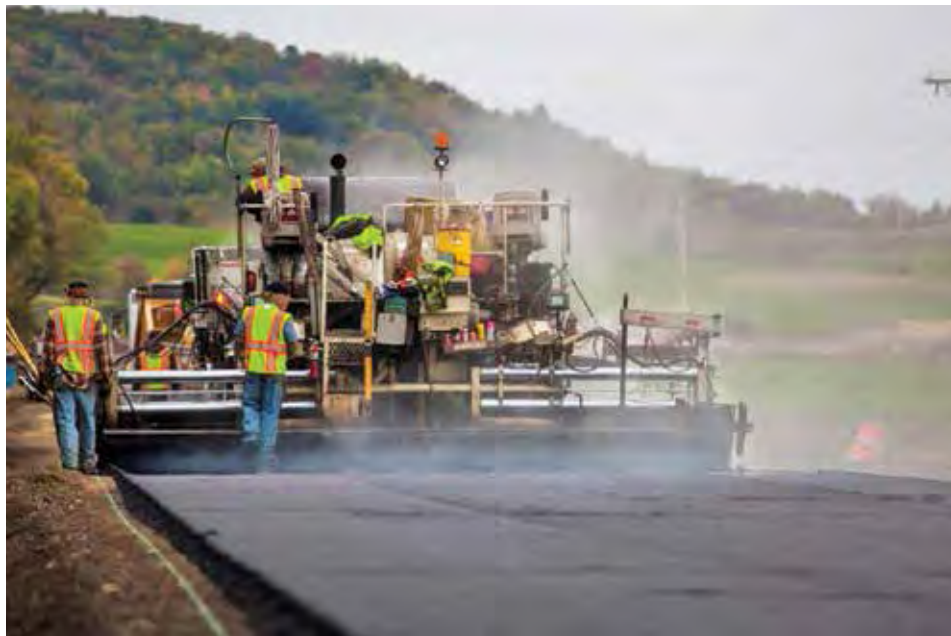
Photo courtesy of Nick Radloff, Mathy Construction
