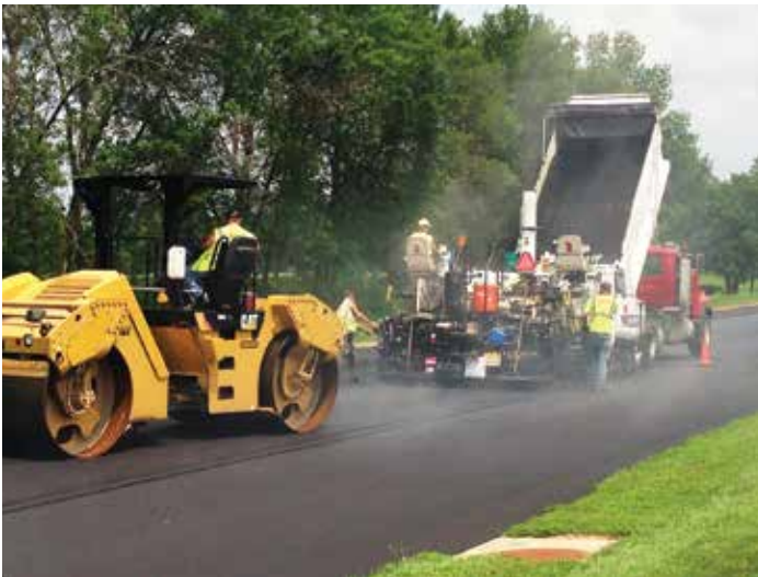
Aspro Inc. paving the Asphalt Interlayer for the City of Waterloo.
