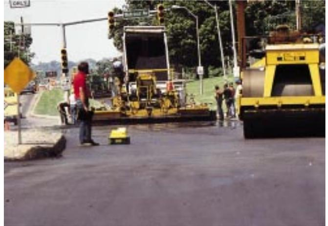
Compaction Testing-Nuclear Gauge
