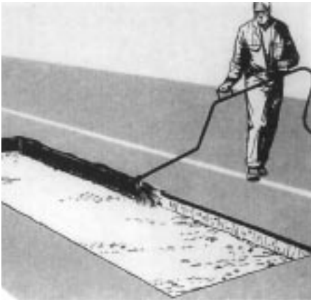
Applying Tack Coat
