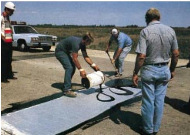
An example of a possible use would be as a spot application on asphalt pavement sections that show signs of alligator cracking related to a weakened subgrade condition. Fabric would be placed just before the asphalt concrete
