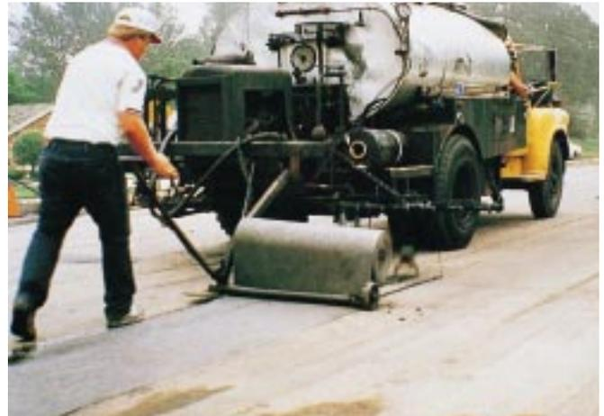
Experimental studies of fabric applications in Iowa have not been conclusive. Early reflective cracking may be delayed through the use of fabric in many cases, especially over a nonworking joint. Also, where water in the pavement structure is a potential problem, fabric can aid in the development of a waterproof membrane.
