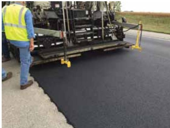
to be Friction Type 4 for non-interstates and Friction Type 2 for interstate work. The use of RAP was not allowed. For construction, HPTO requires the use of a “trackless tack”, a temperature of 60° F and rising, and a Class II compaction with a steel drum roller.
