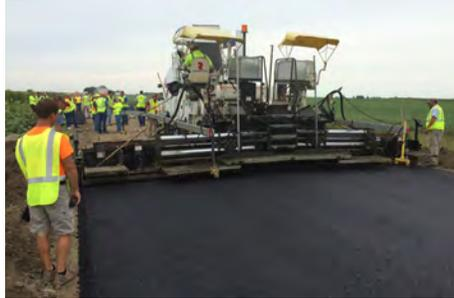
trimmed with a 12 foot milling machine to achieve desired slope and grade. The Open House highlighted the strength of the full-depth reclamation (FDR) process in creating a stable and homogenous platform to pave upon. The project was
