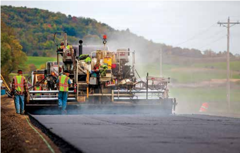
Photograph by Nick Radloff, Mathy Construction Co.
