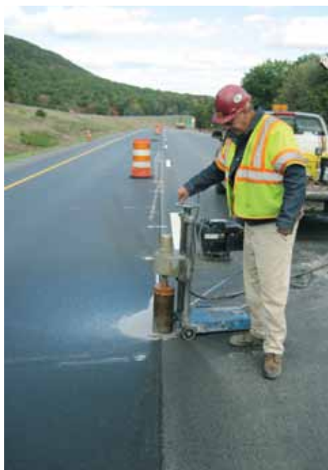
Cutting a Density Core on a Vertical Centerline Joint
