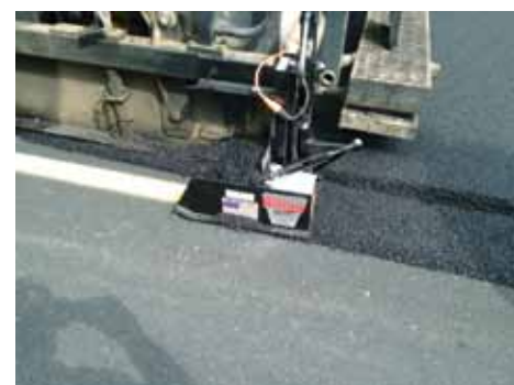
A vibratory plate attachment compacts the taper in a notched-wedge joint.
