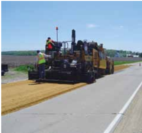
Mathy Construction places Rock Interlayer on Scott Co. Y4E in 2011.
