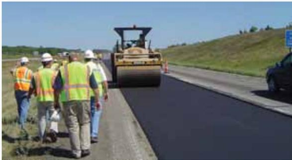
Heartland Asphalt paving Asphalt Interlayer on I-35.
