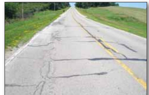
SE 32nd prior to rehabilitation
