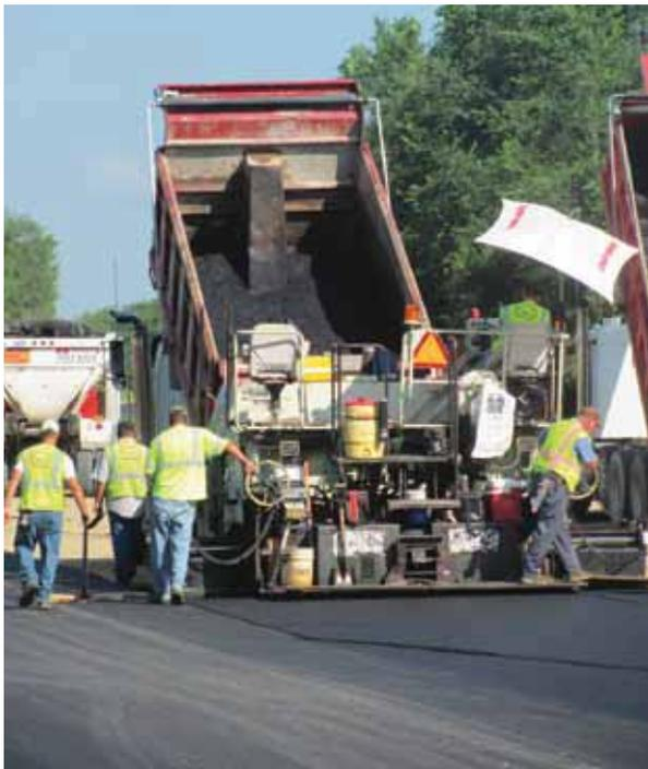
a foaming process or chemical additive. The benefits from using warm mix asphalt are remarkable: lower fuel consumption, better work environment, increased hauling distances, and an extended paving season.
